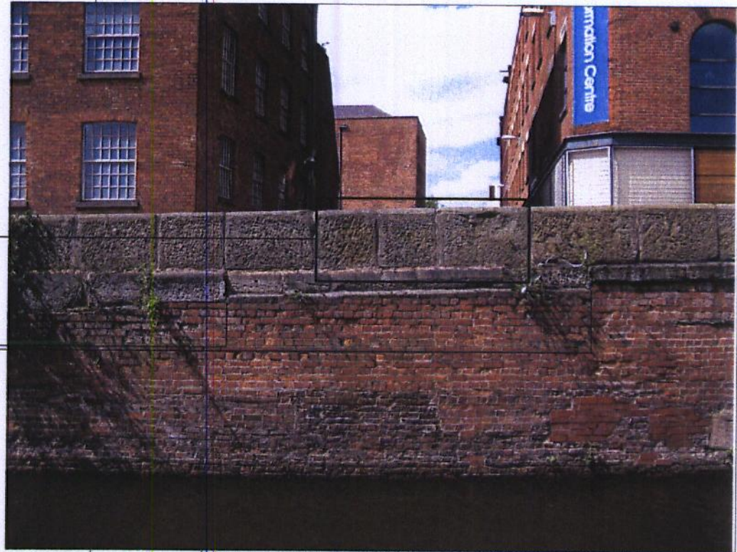
View of Redhill Street Canal Wall
